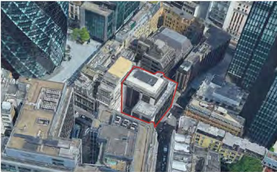
Figure 1 – Image from Design and Access Statement by Stiff & Trevillion showing the location of the proposed development with Valiant House and Bevis Marks Synagogue to the north
